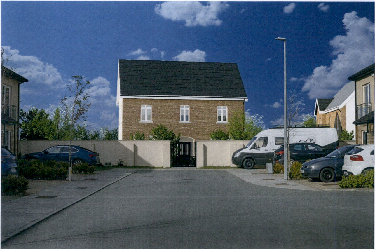
Figure 1 Existing gate with permitted development beyond viewed from Silken Park
