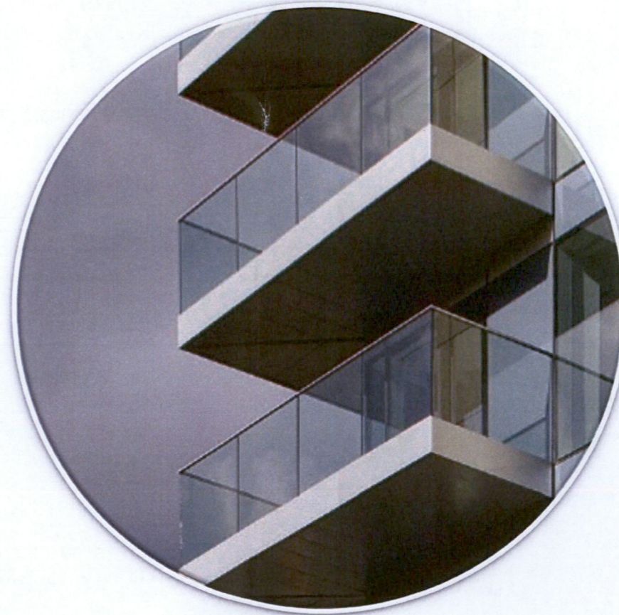
Apartment Balcony Glass Balustrade
