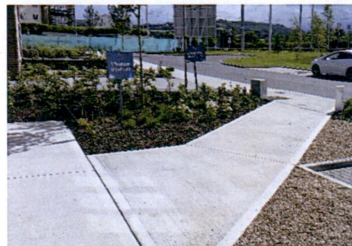
Brushed Concrete to build out edges
