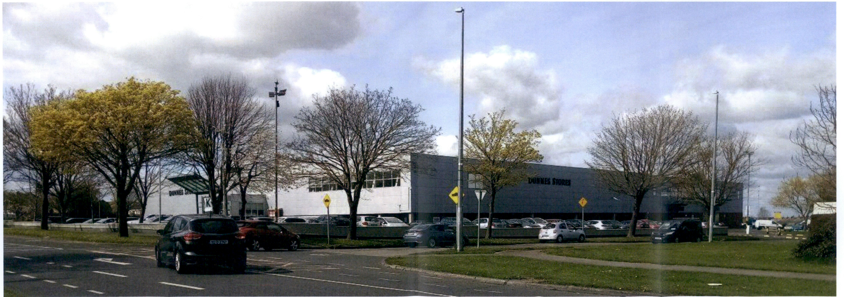
Existing Street view No.1 – Mayberry Road
