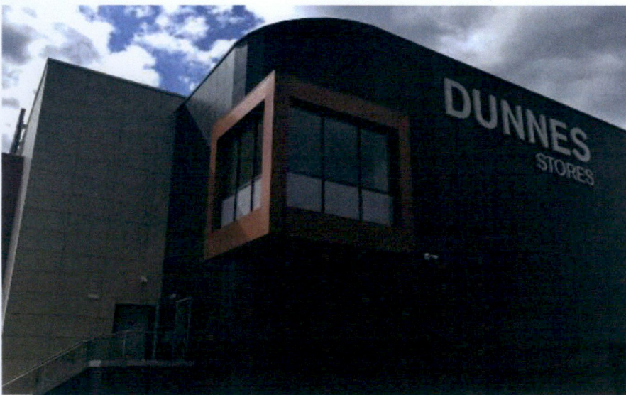
Sample of dark ceramic cladding with copper window framing and white signage
