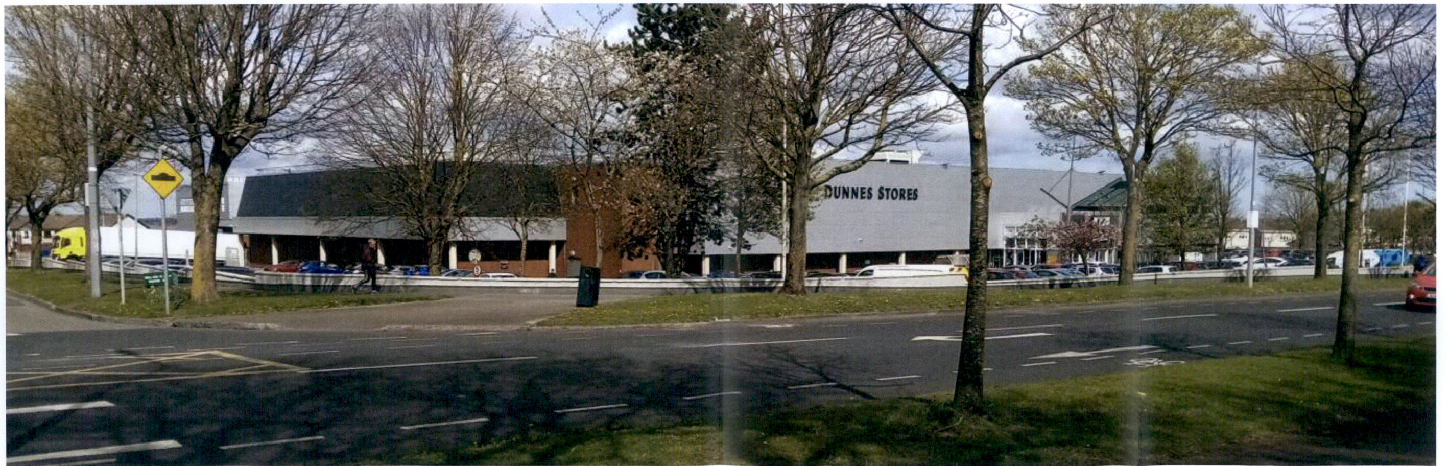
Existing Street view No.2 – Mayberry Road
