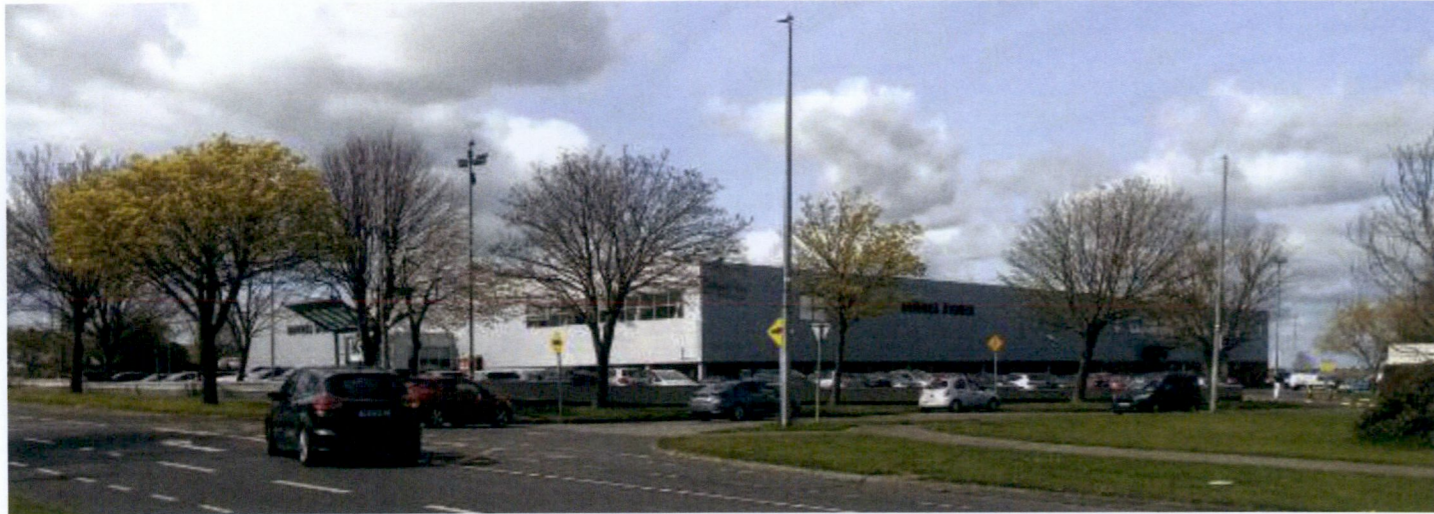
Existing External View 1
