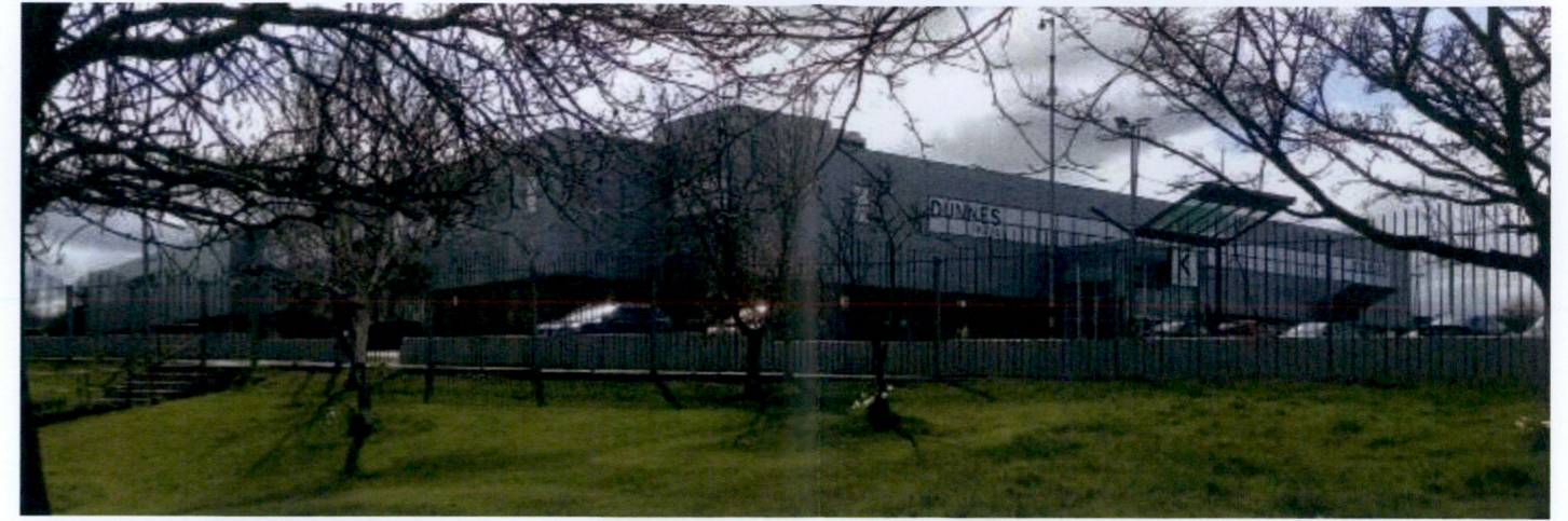
Existing External View 3
