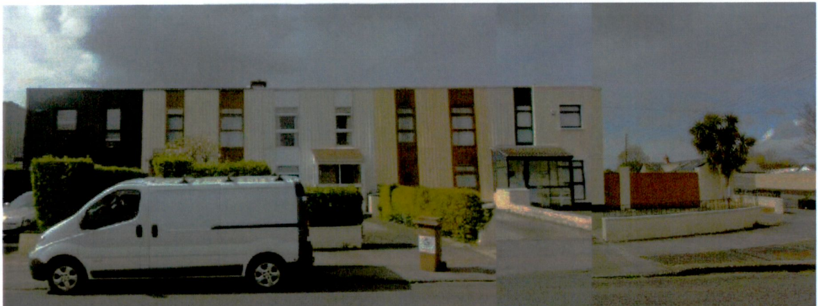
• Photomontage of East Elevation of No. 20-22 Tara Hill Road. No. 24 to Right.
