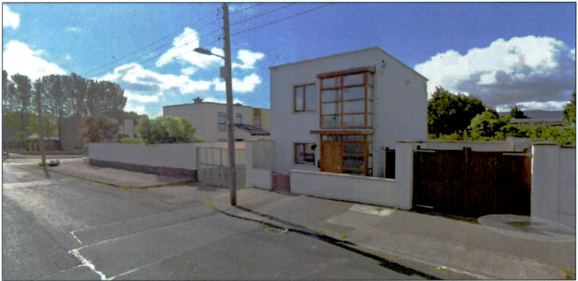
• No. 22A on right of image behind site, and our site to left of image, with rear lane access gate behind pole.
