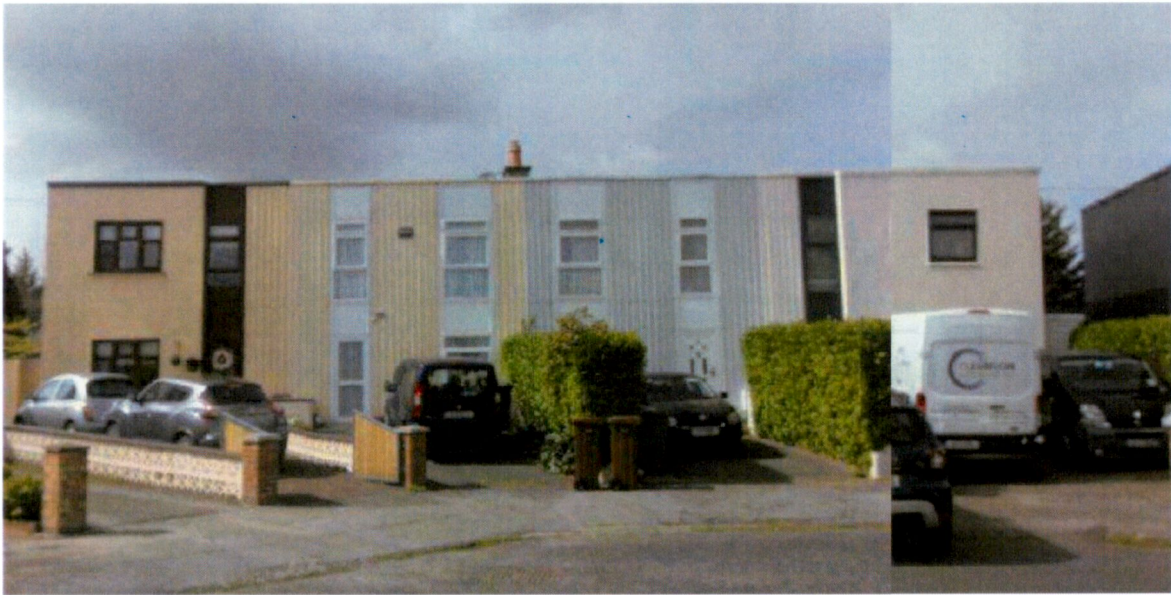
• East Elevation of No.16-19 Tara Hill Road.
