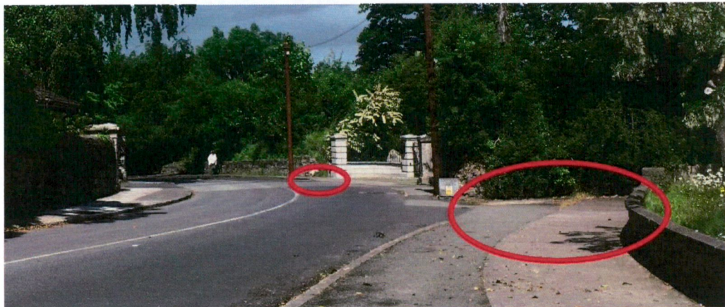
Figure 6 Footpaths at entrance
