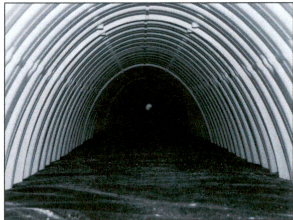
Looking down the Isolator Row.
