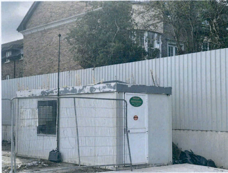
Pic 1: Setup at NML1 adjacent No. 24 Brownsbarn Wood front elevation.
