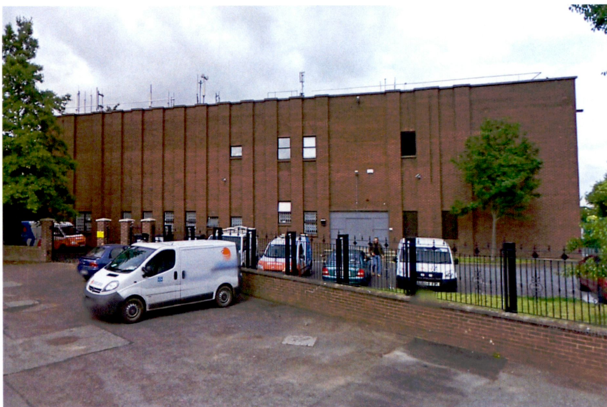
Figure 1: Existing Rooftop Site
