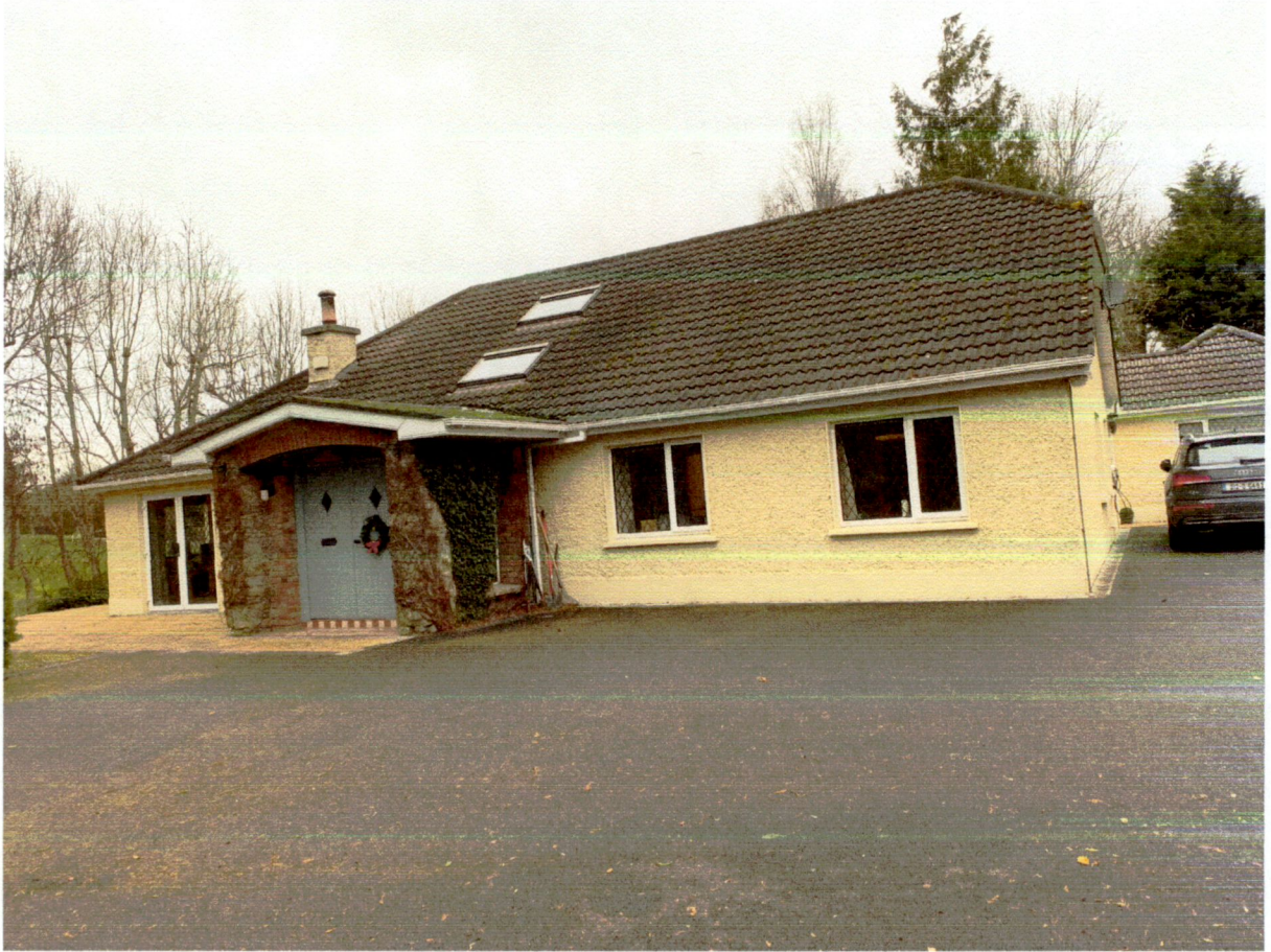
THE EXISTING DWELLING
