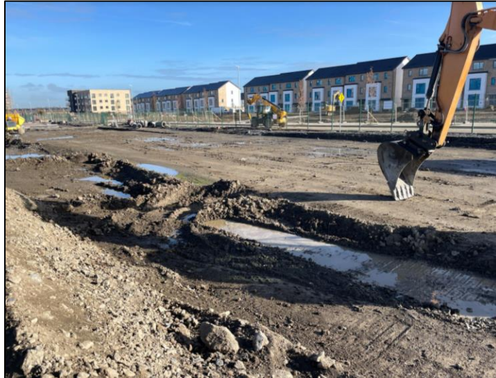
Plate 2: Excavated areas at the east of the site
