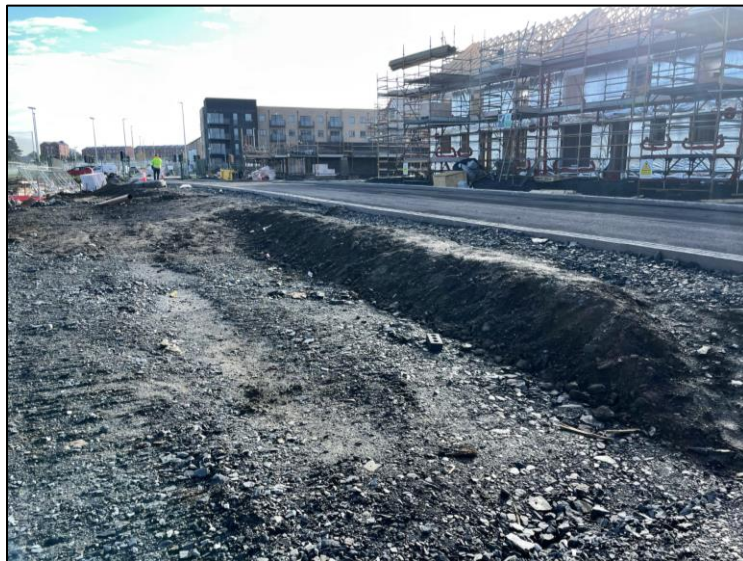
Plate 4: Exposed baulks at the north of the site, looking southeast
