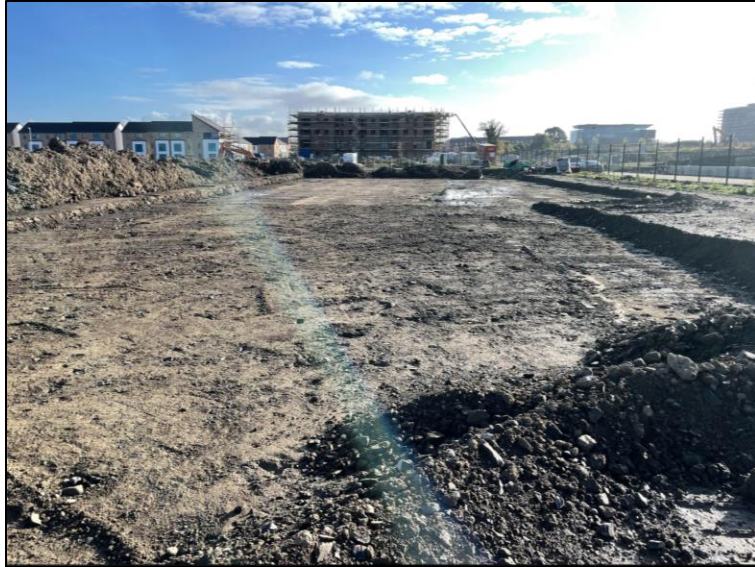
Plate 3: Looking east at excavated areas at the south of the site
