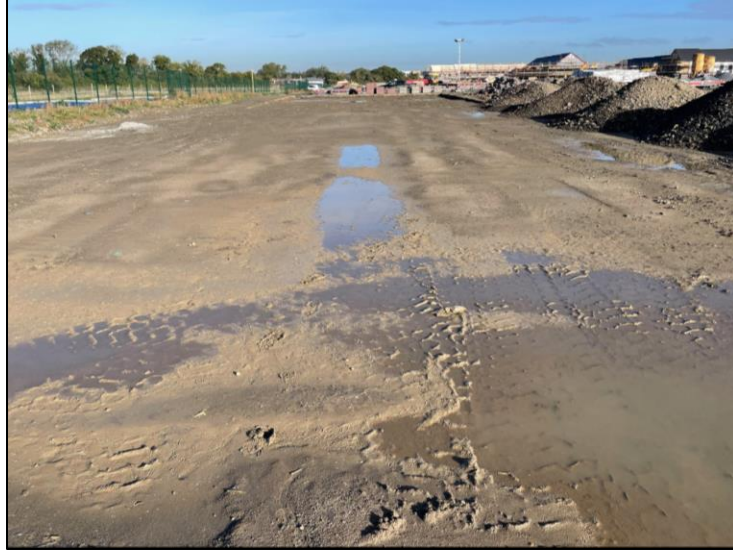
Plate 1: Looking south over excavated areas at the south of the site
