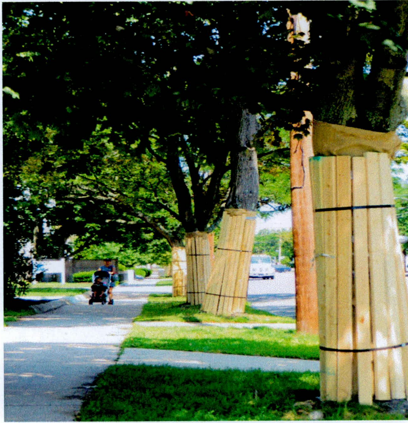
Figure 4. Displays the protective wrapping to placed on the retained trees to avoid mechanical damage to the main stems.
