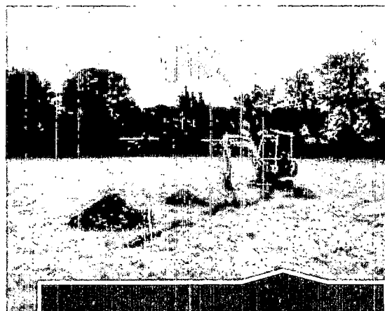
Site during testing. Brownsbarn - 24-08-2022
