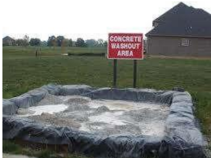
Figure 5-4 Example of temporary concrete washout area
