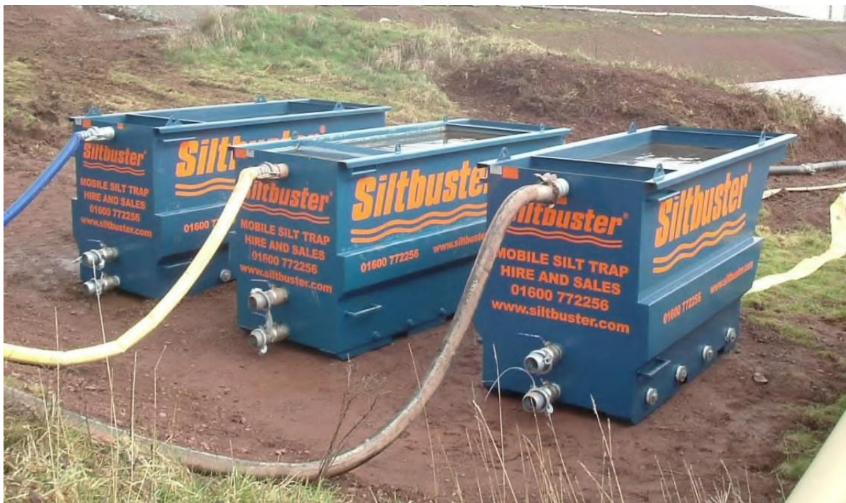
Figure 5-3 Temporary site settlement tanks (Source: Siltbuster)
