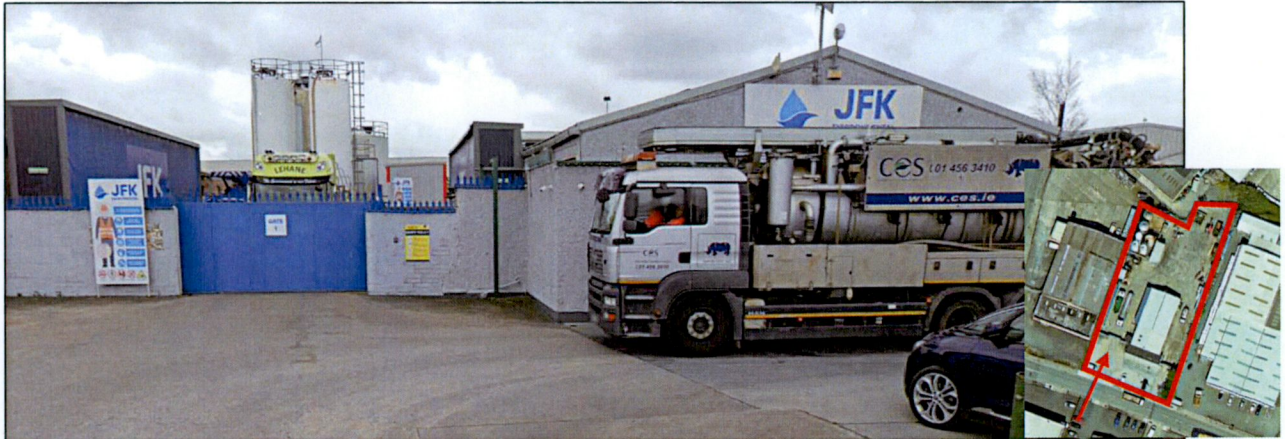
Figure 2.4: View of Subject Site from JFK Road (Arrow in Red Indicates the Camera Direction)
