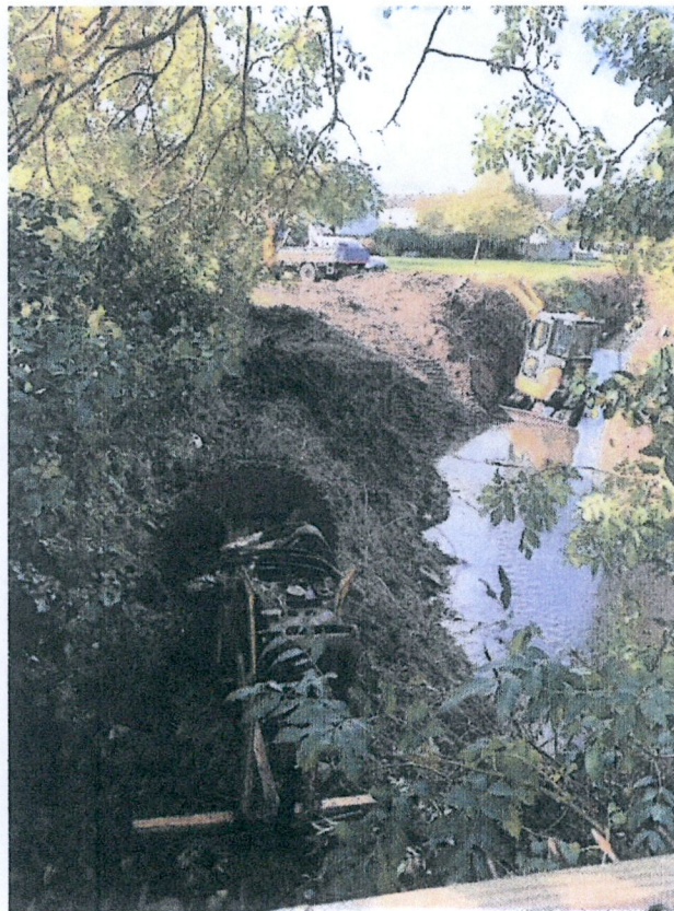
8) View over fence looking West at cleared vegetation from riverbank
