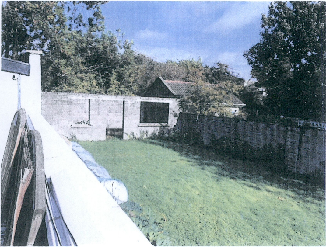
3) Front/south elevation of existing adjoining blockwork sheds to no.7 & no.9
