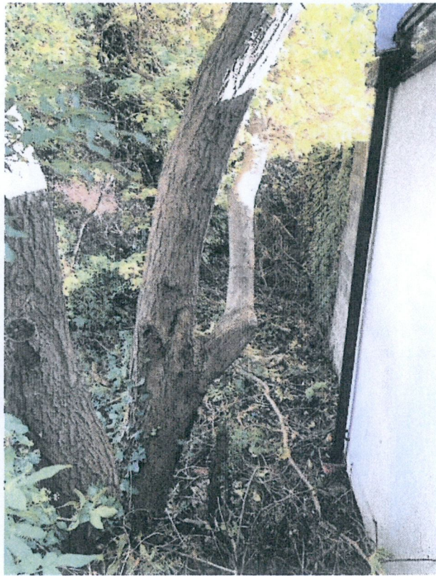
7) View of remaining rear elevation of garden room & retained tree
