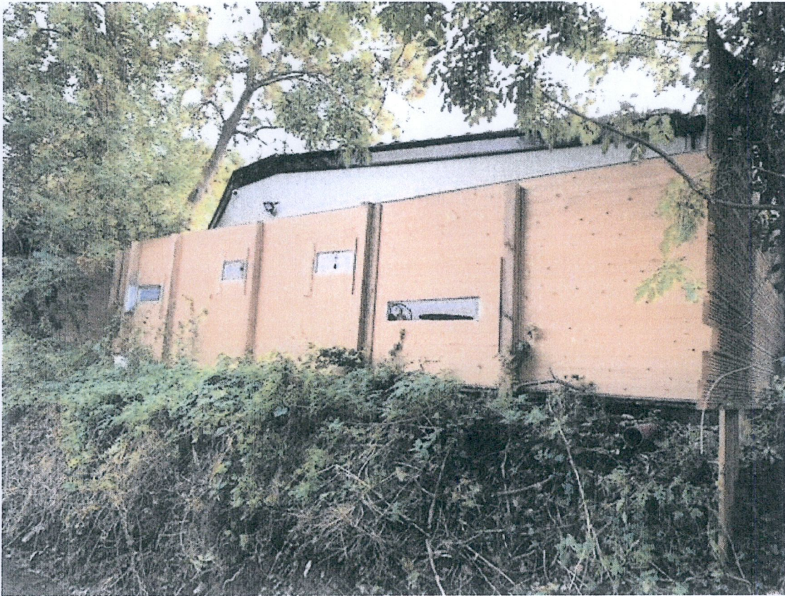
9) View of Rear boundary fence & part rear elevation from riverbed
