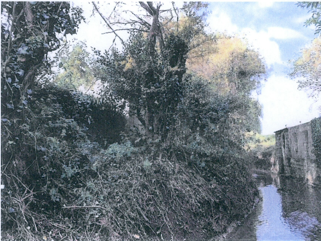
18) View back upstream at cleared vegetation from riverbank (looking west)
