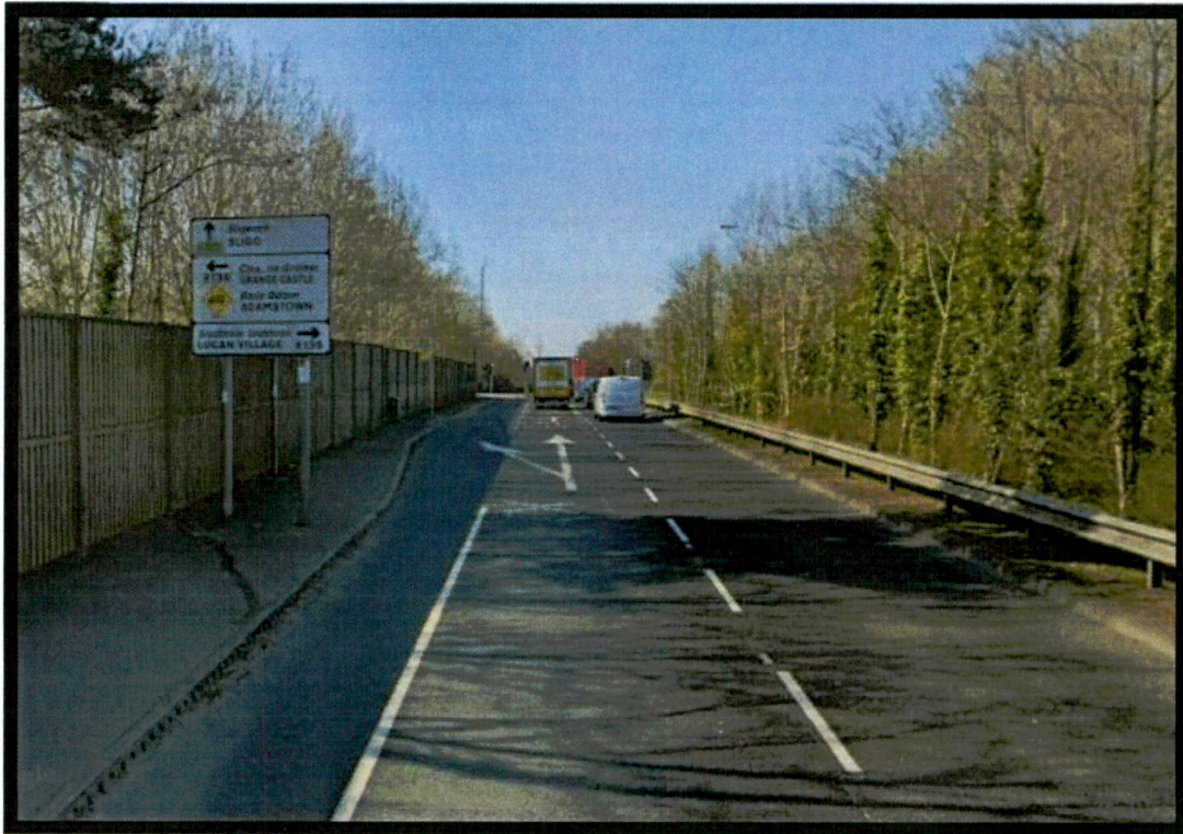
Figure 2.4 – Service Road/Slip Road Westbound Approach to Junction #3
