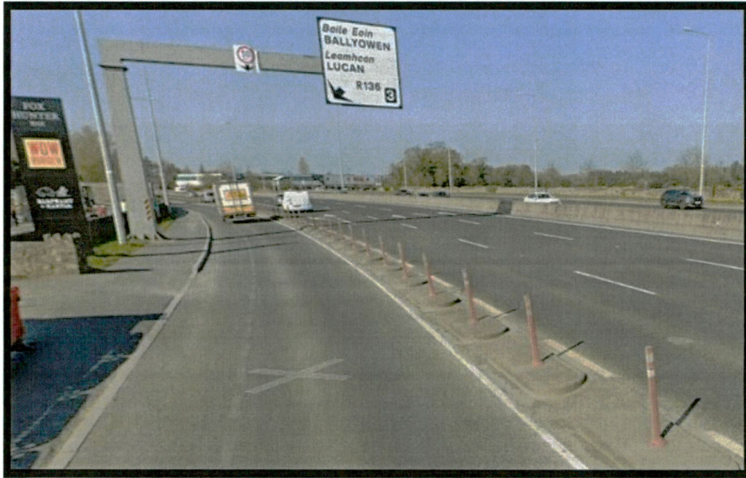
Figure 2.1 – Existing Eastern Vehicular Access to Service Road
