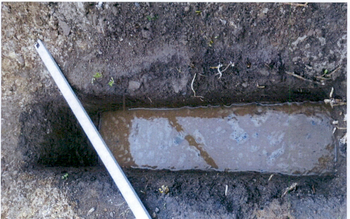
Pit during test
