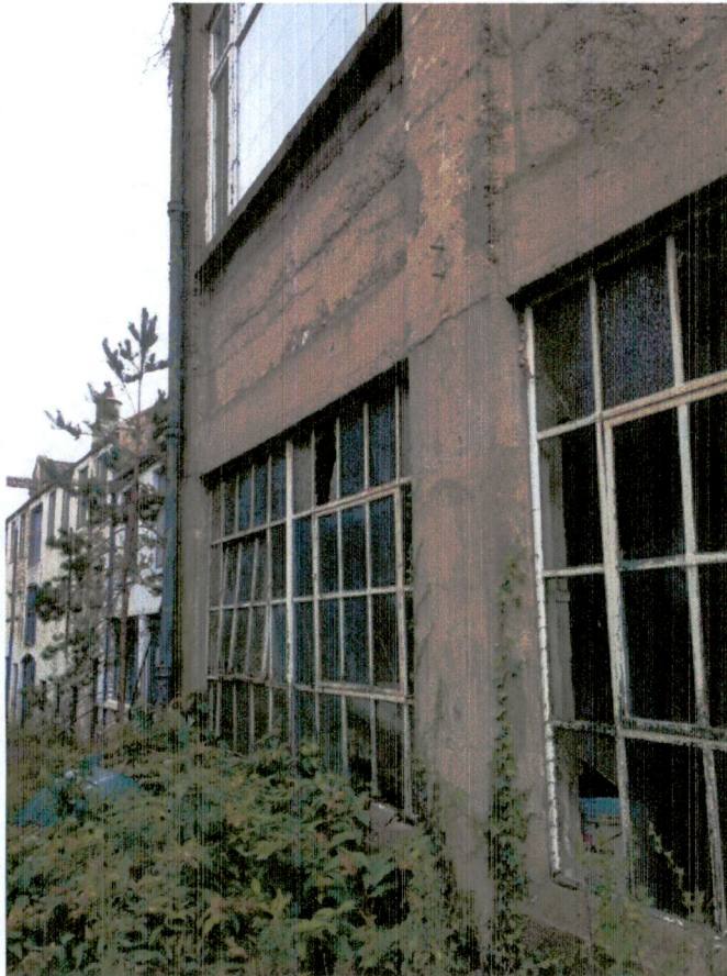
Fig.11 Example of boardmarked concrete externally
