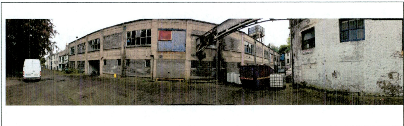
Fig. Building C
