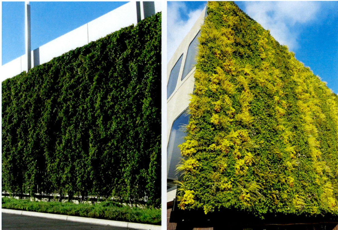
Green façade system utilising climbers on wire trellis (left) and alternative cellular 'living wall' system to right
