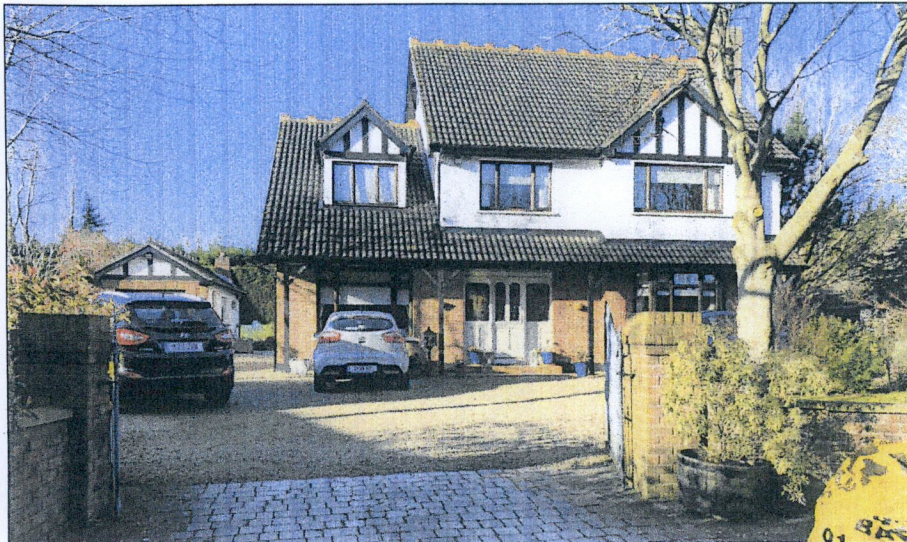
Front elevation and garage to be demolished of The Muddies from private laneway
