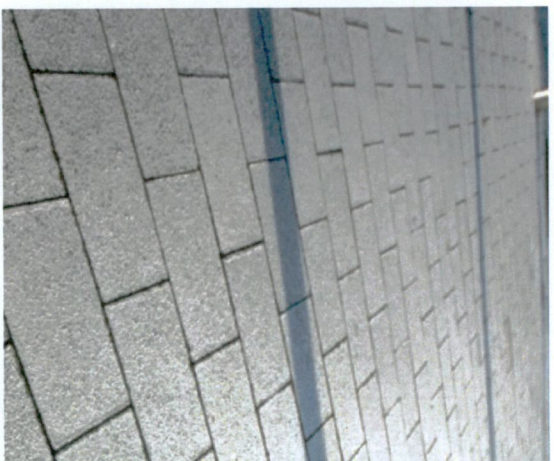
Core building entrance paving - Silver granite PCC pavlours
