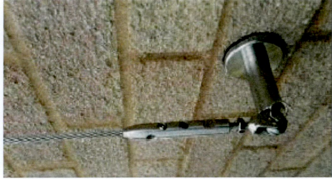
Jaw tensioner attached to pro-eye fitting
