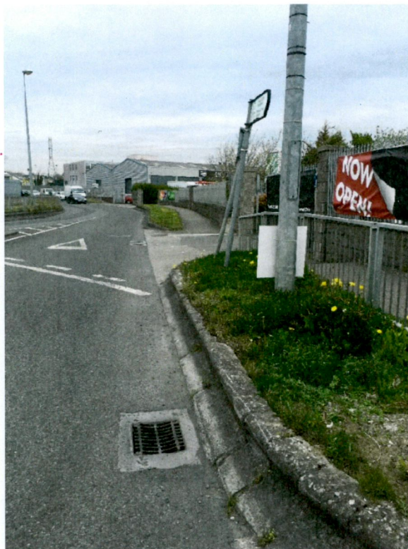
View from Cookstown Road/ Second Avenue junction, a scene typical throughout the Cookstown Estate, with large 'Kassel' type kerbs, poorly maintained grass verges and pedestrian 'crash' barriers.
