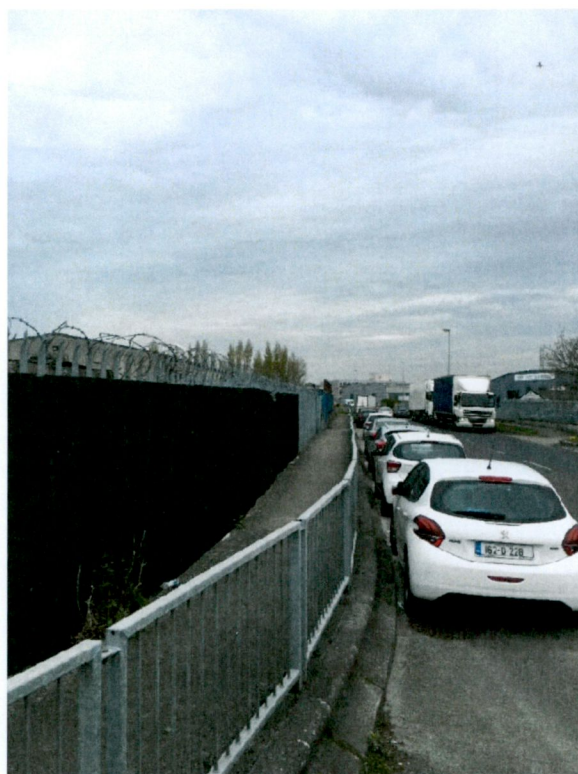
View looking north from Cookstown Road/ Third Avenue junction towards subject site. Large 'Kassel' type kerbing, crash barriers and boundary treatments of palisade fence and razor wire.
