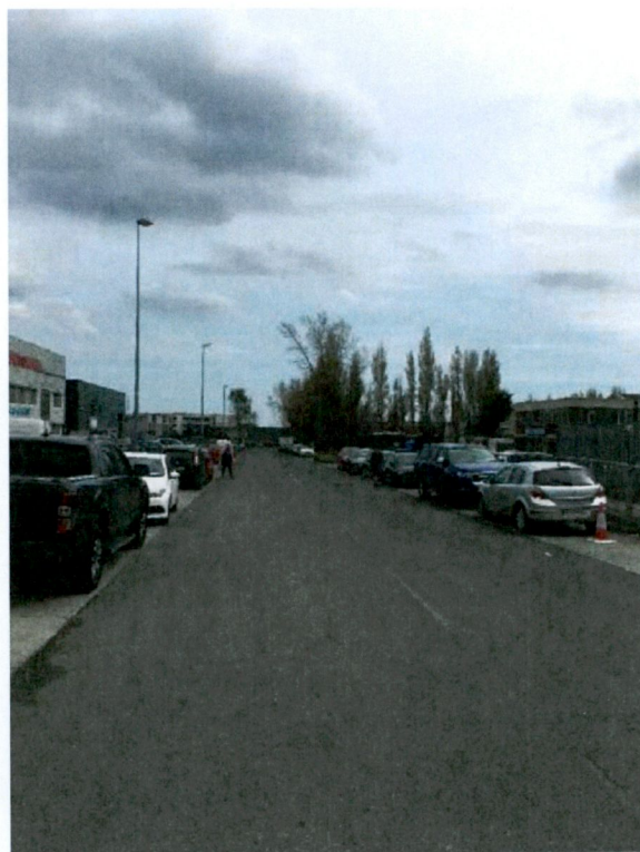
View east along 1 st Avenue towards the subject site. In-situ concrete parking bays, asphalt road surface with galvanised steel pedestrian barriers.
