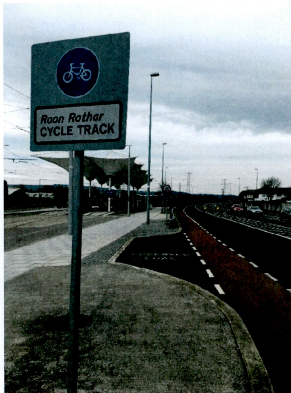
View west along Bóthar Katharine Tynan: The Belgard Luas stop is visible to the left of view. The stop acts as a transfer hub serving the Redline links into the city centre from Tallaght and the spur to Saggart.
