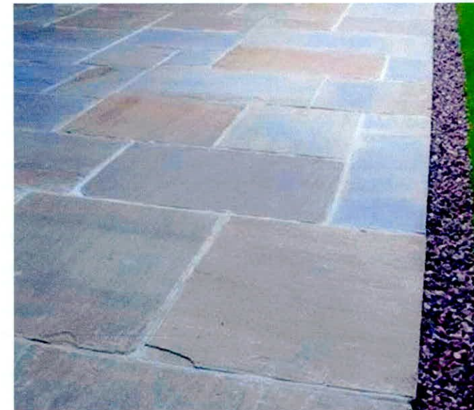
Fig: 24 Riven face Yorkshire stone flag paving to terraces
