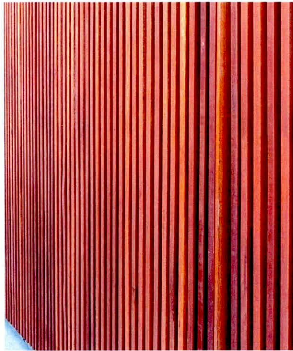
Fig: 21 Hardwood batten hardwood cladding sample image
