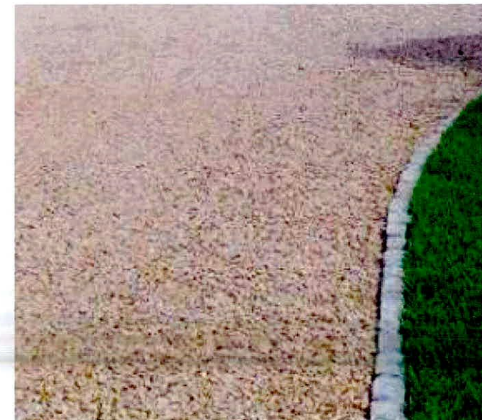
Fig: 25 Compact pea gravel permeable driveway
