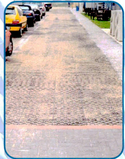
Car Park Infiltration Area.
