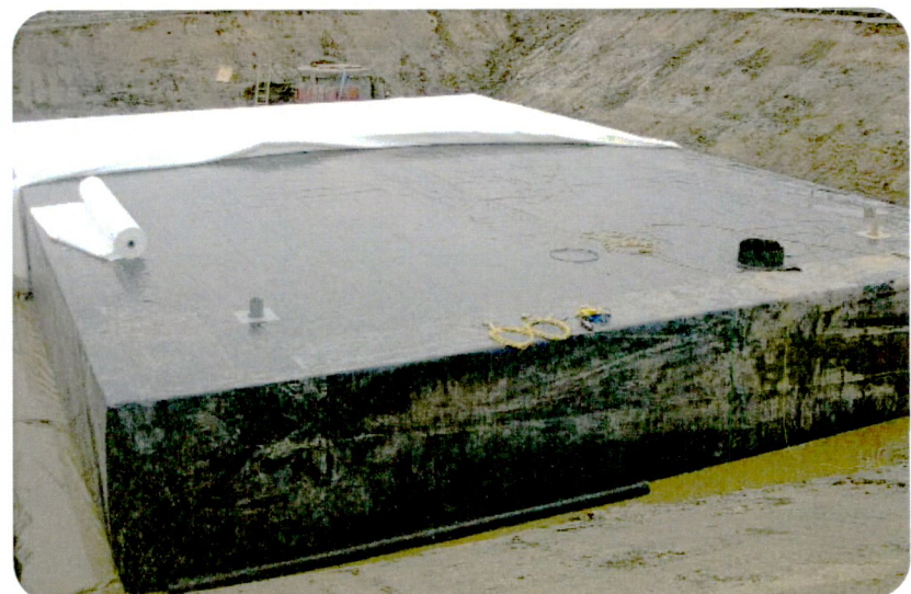
2mts deep tank with 3mts cover
