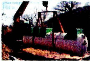
► Each WWT Plant is constructed of lightweight SMC and is easy to manoeuvre which simplifies the installation process.
