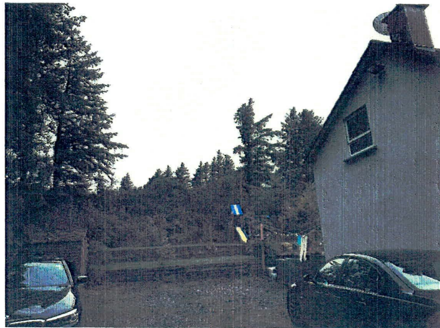
View of Side of House at proposed Extension
