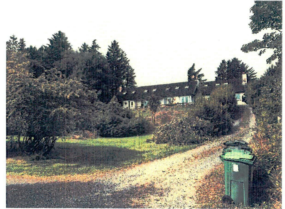
View of House From Emtrance Gate
