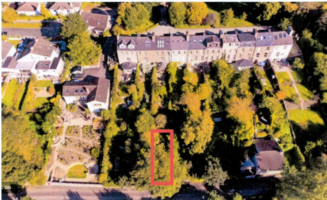
AERIEL VIEW OF No1 THE CRESCENT LUCAN (MEWS SITE OUTLINED IN RED)
