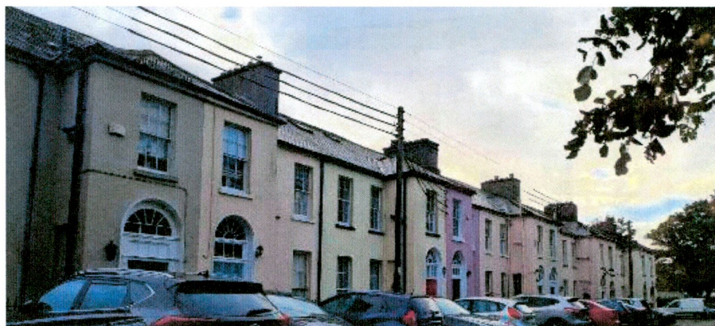
Contextual view of the front elevation – The Crescent Lucan
