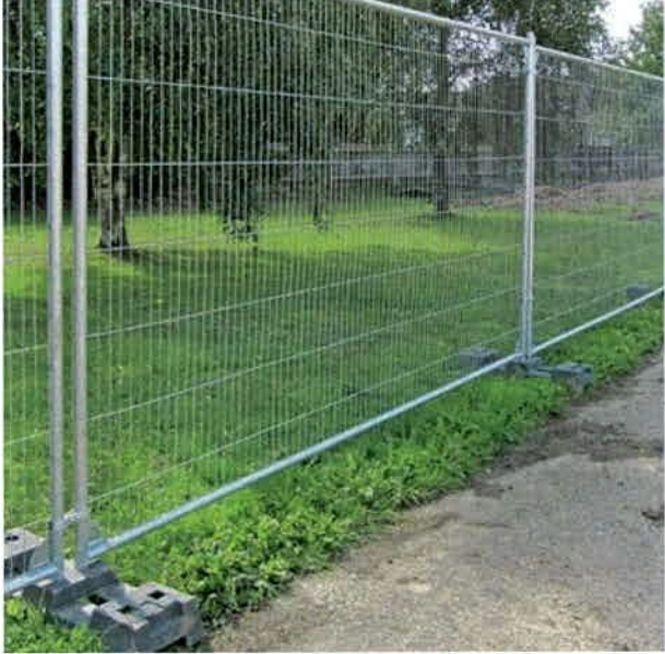
Block and Mesh Fence
