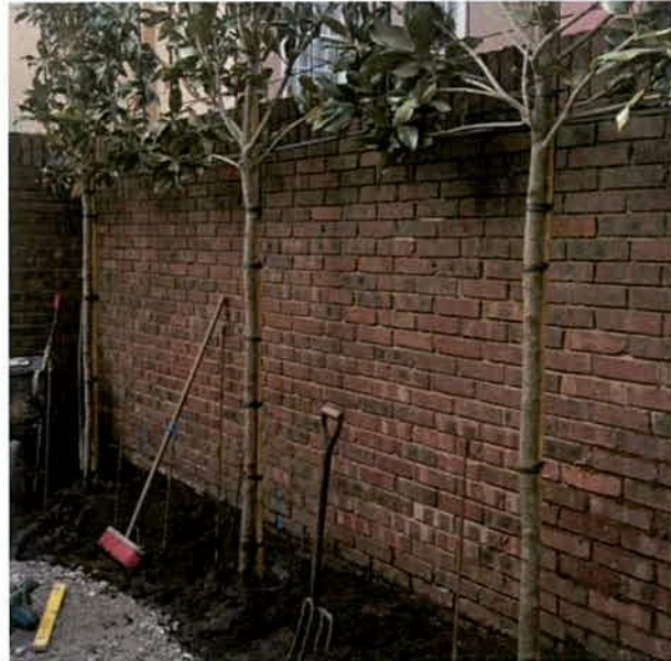
Block Garden Wall - Not suitable for use along hedgerow - Colour of brick refer to architect's specification
