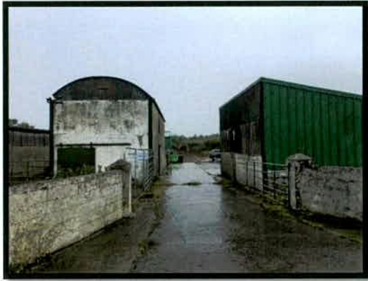
Structure 1 and Structures 3 – External
