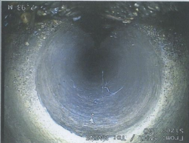
Dimensions of drain/sewer changes to 100mm
