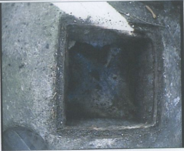
Manhole / Access Point: FAJ1 Internal
