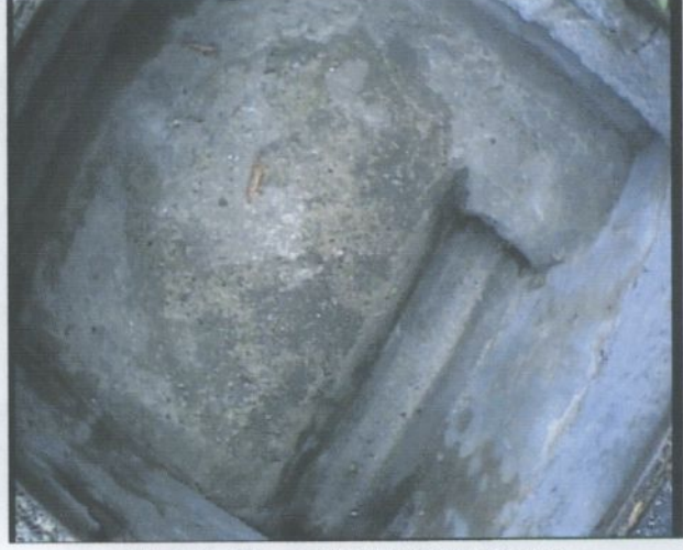
Manhole / Access Point: EX SMH Internal
