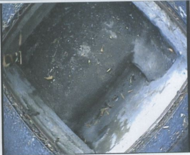
Manhole / Access Point: SMH1 Internal
