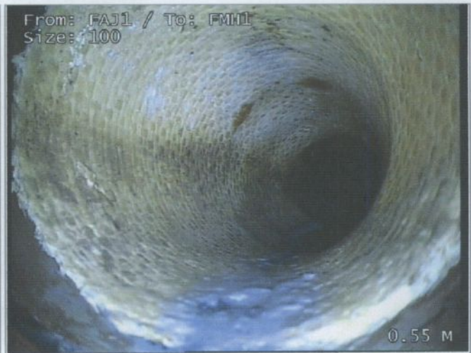
General photograph taken at this point - Remark: PART LINER INSTALLED
