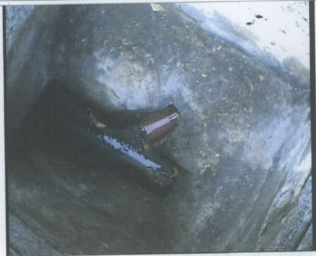
Manhole / Access Point: FMH1 Internal
