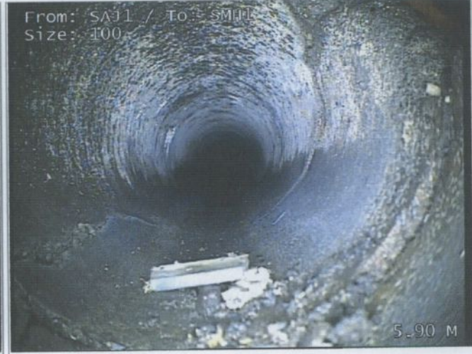
Fracture spiral from 8 to 1 o'clock
