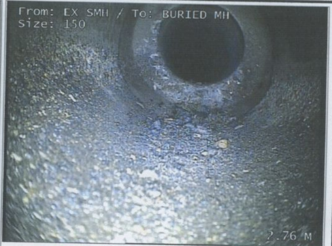
Dimensions of drain/sewer changes to 100mm
