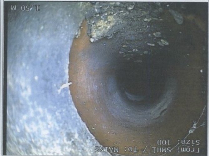
Material of drain/sewer changes to vitrified clay at this point
