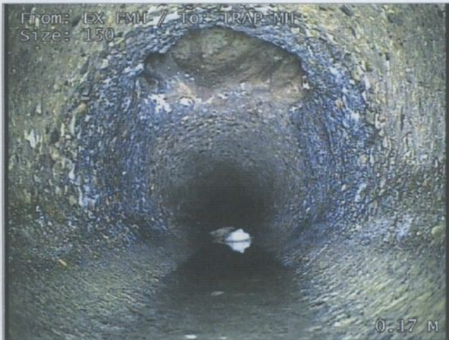
Connection other than junction at 12 o'clock, diameter 100mm
