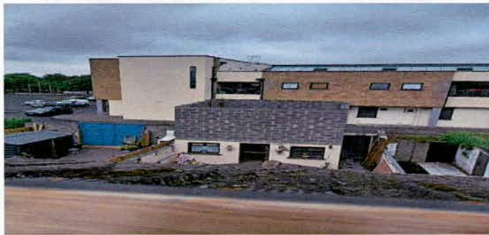
VIEW FROM No. 38 SHOWING WALLS ERECTED AT FIRST FLOOR.
