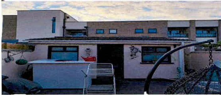
EXISTING SHED BEFORE WALLS WHERE BUILT AT FIRST FLOOR
