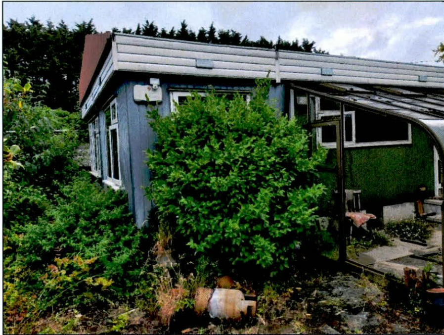
Plate 2 Side (west) elevation of vacated bungalow, facing north.
