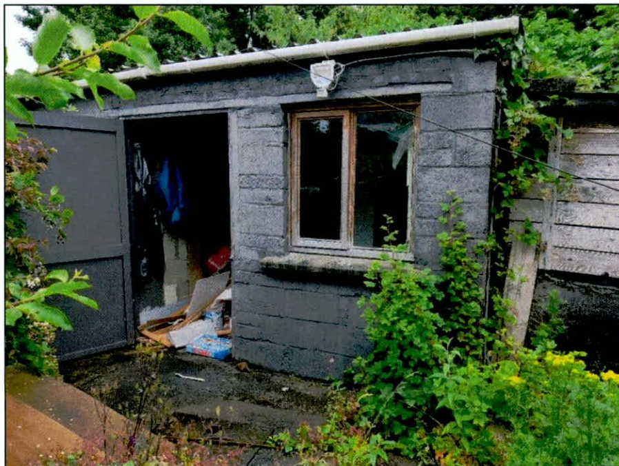
Plate 3 Rear shed to north-western corner, facing north-west.
