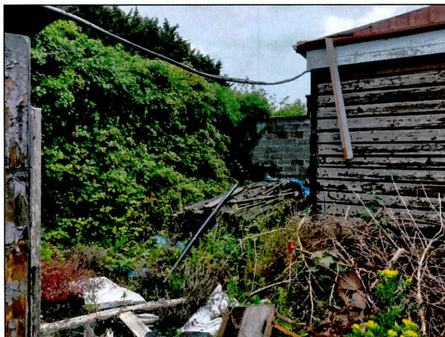
Plate 5 View of overgrown rear (northern) boundary wall, facing east-northeast.
