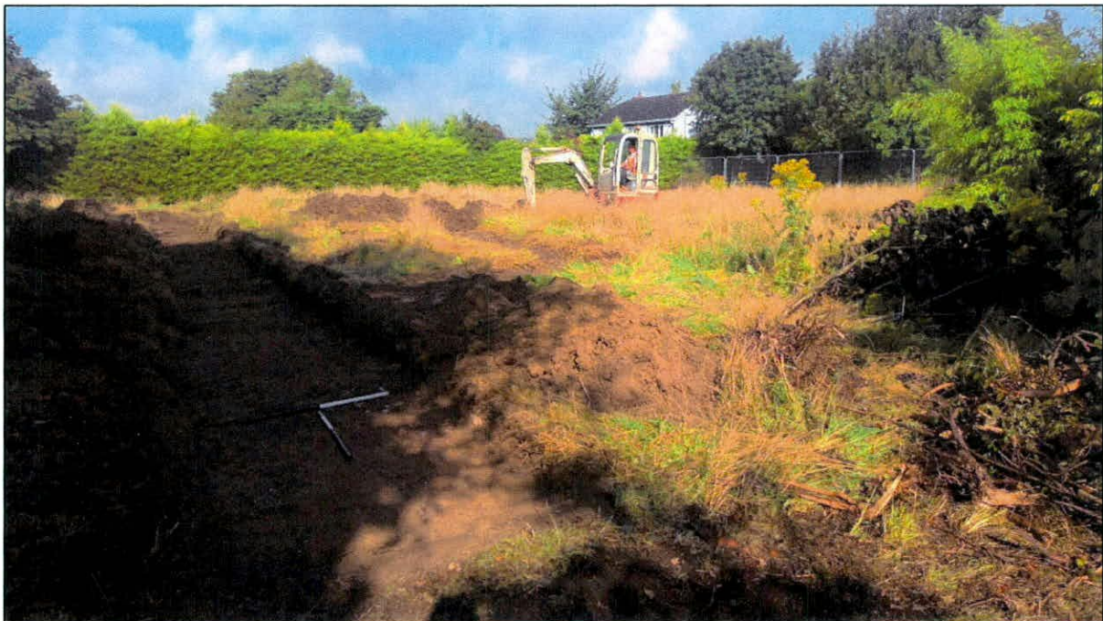
Plate 1: Looking northwest during excavation of test trenches
