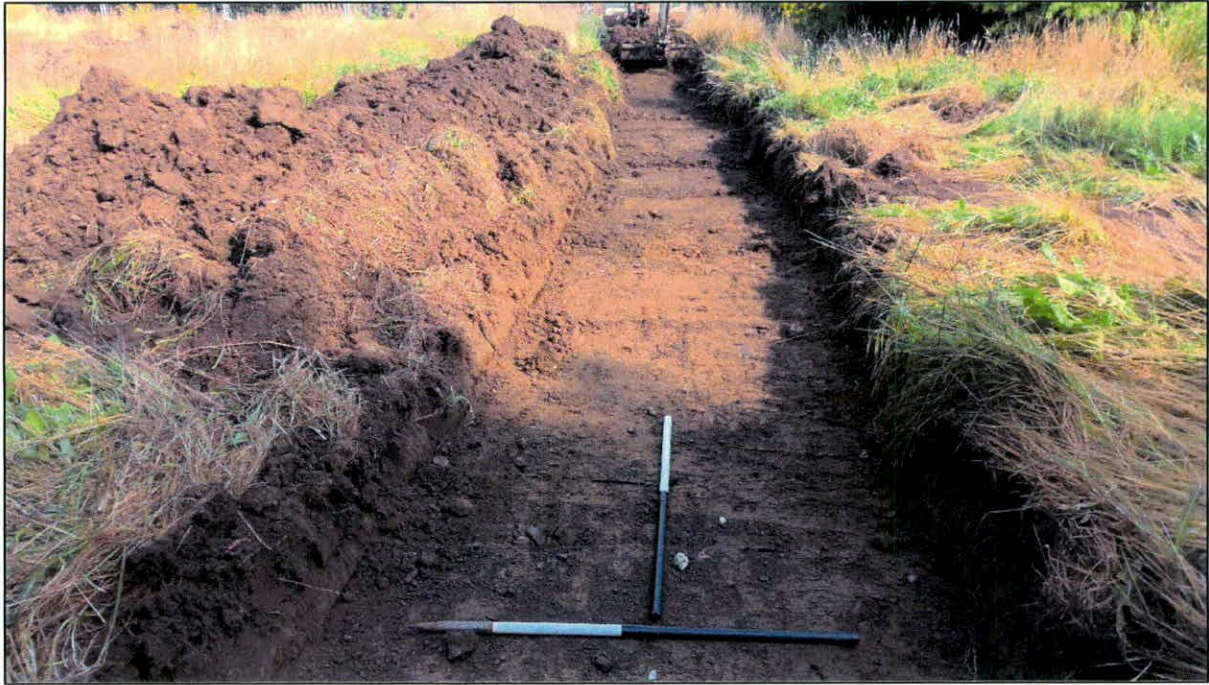
Plate 4: Test trench 4, during excavation, looking north
