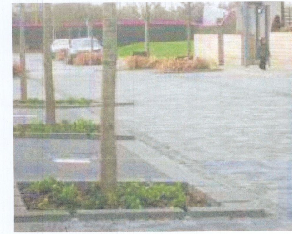
FIGURE 19.16: EXAMPLE OF INLETS TO ALLOW SURFACE WATER RUNOFF TO INFILTRATE INTO TREE PITS. TAKEN FROM CIRIA REPORT C753 THE SUDS MANUAL.
