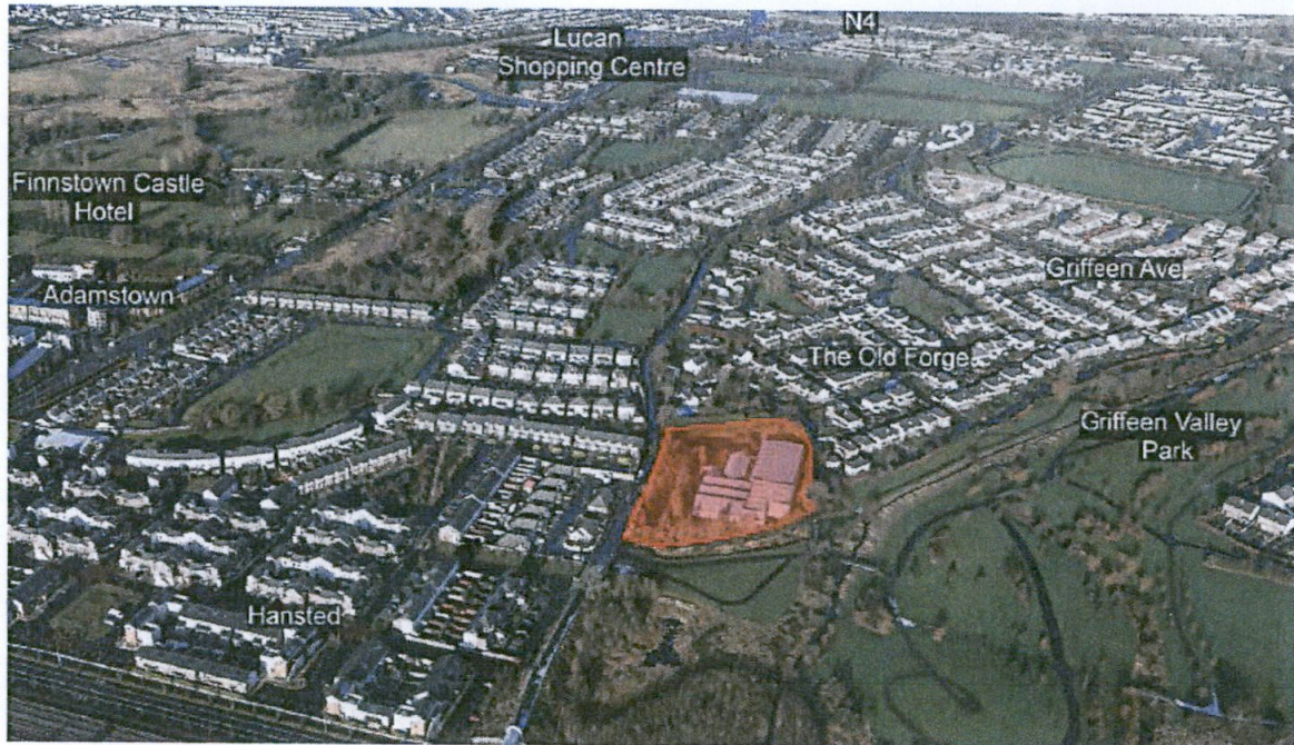
Figure 1: Aerial View of Site (showing previous factory building on site)
