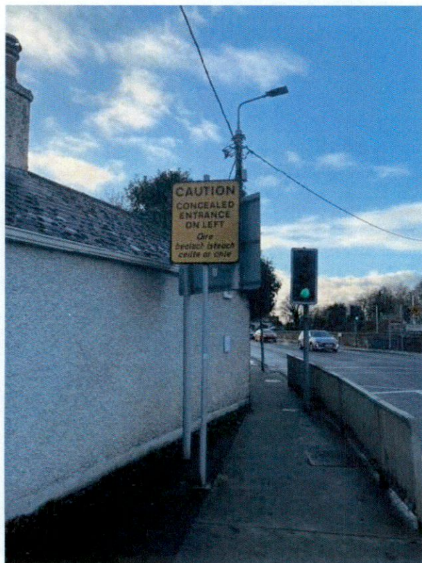
Figure 2. Shows the path on the northwest corner of the proposed development. This is a pinch point on the pedestrian walkway with insufficient width for two people to pass alongside each other
