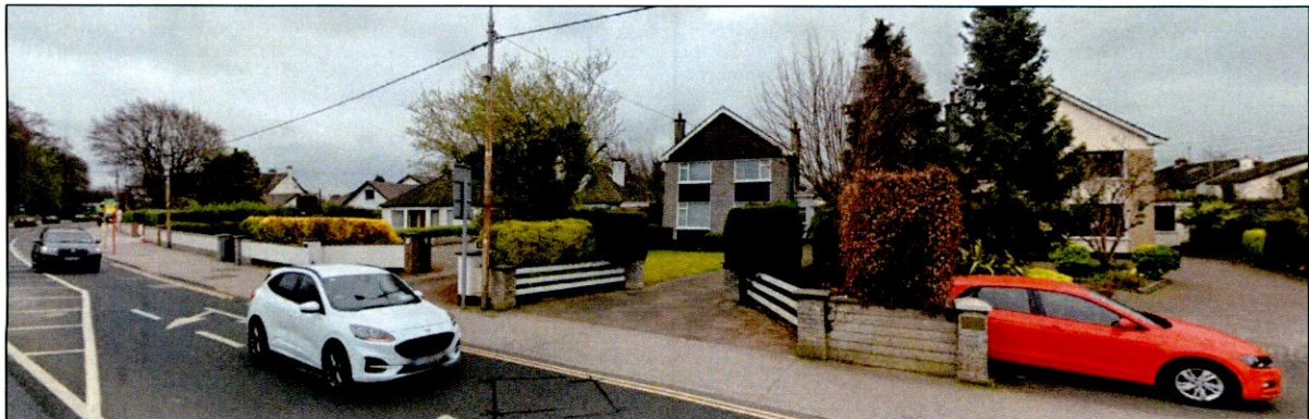
Figure 18.0 Existing streetscape of the Lucan Road displaying the existing built form.
