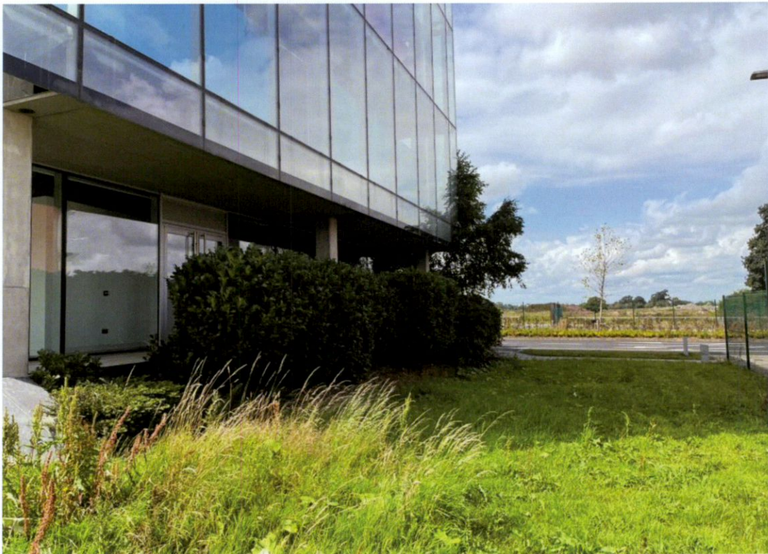
Photo 4: View of the shrubs (S566) located along the northern side of the building.
