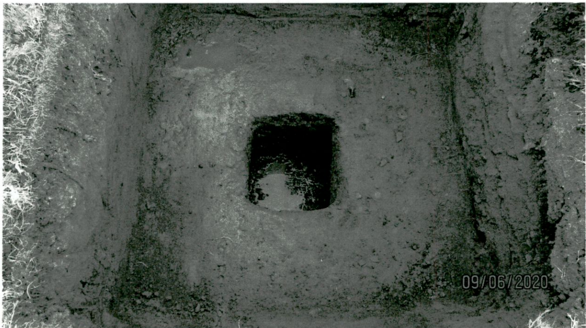
Photo No 8: T-Test Hole No 2
