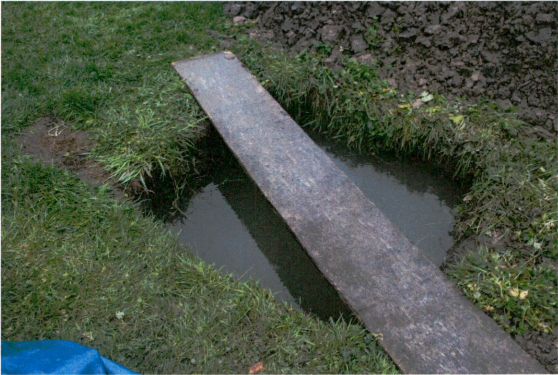
PHOTOGRAPH NO.1: TRIAL PIT
