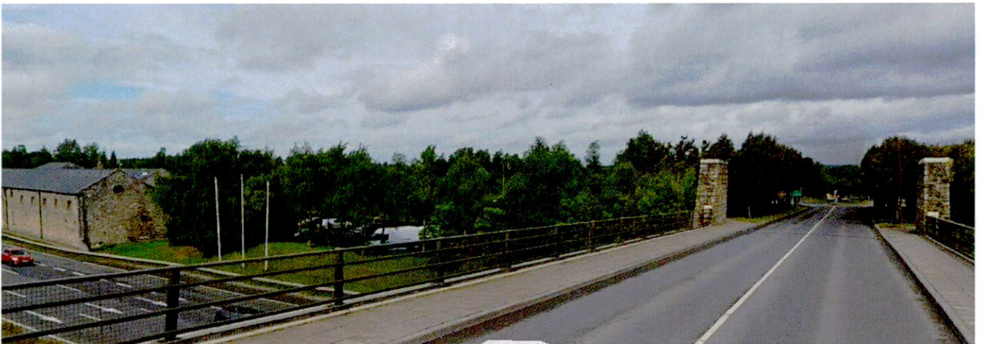
Figure 5: Image From Street level on overpass at Exit 3 on the N7 (building screened by trees)
