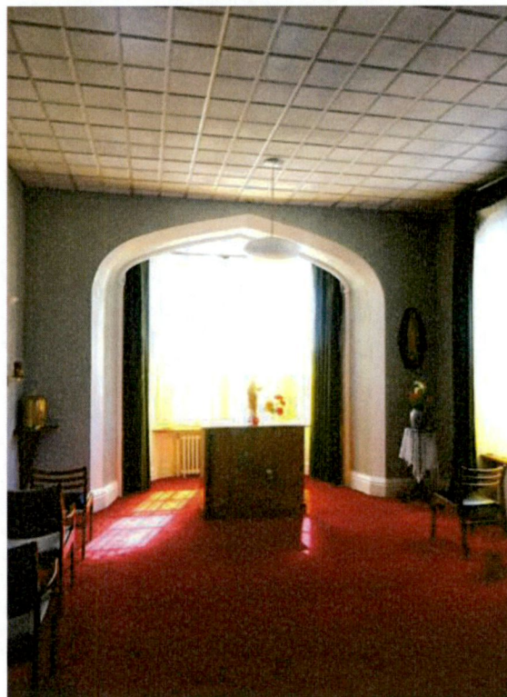
View above G12 of the former living room located at the junction of the eastern and southern wings with modern dropped ceiling and presently used as a private chapel. The room retains good window joinery, likely cornice-work above dropped ceiling and an original chimneypiece.
