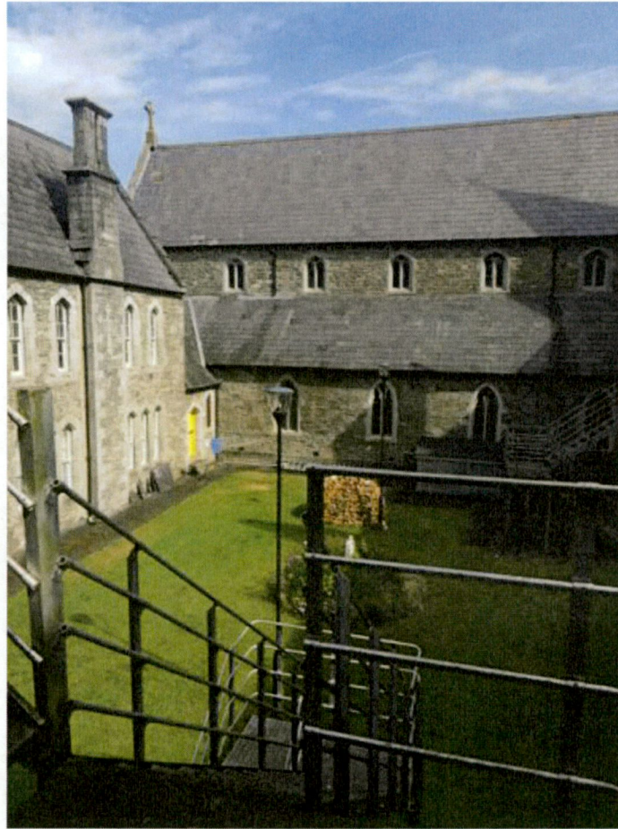
View from fire escape towards north eastern corner of internal courtyard (E10) and view E11 below of internal courtyard façade of western wing.
