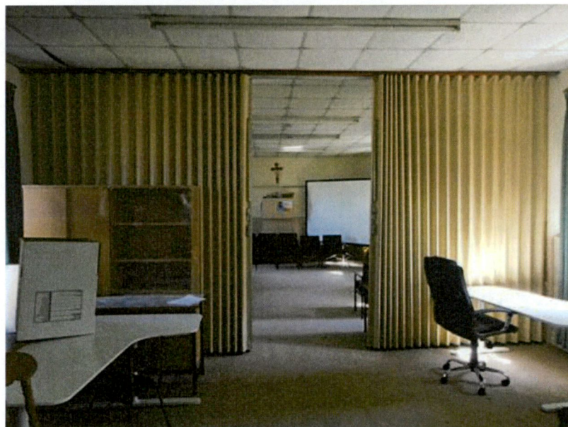
View (above F15 and below F16) of the upper parish meeting room with modern lowered ceiling and original windows and casing extant – otherwise a modernised interior.
