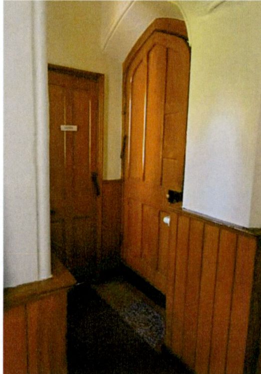
Corridor joinery (above G17) at the junction of the south and east wings is extant, of stained timber and rich and well executed. View (below G18) of the staircase (Stair 01) between the present private chapel and dining room in the south wing with distinctive attenuated finial.
