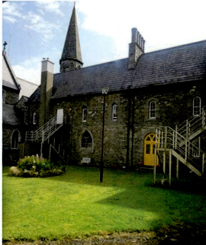
View across the internal courtyard (E9) showing the modern chimney stack and plainer treatment architecturally to the less public internal courtyard facades
