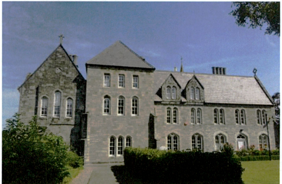
Elevation / view of the south-facing wing E4 : the more utilitarian nature of the three-storey wing is expressed externally with simpler windows and a greater proportion of masonry. The raised wall dormers with paired windows break up the mass of an otherwise large area of plain slate roof.
