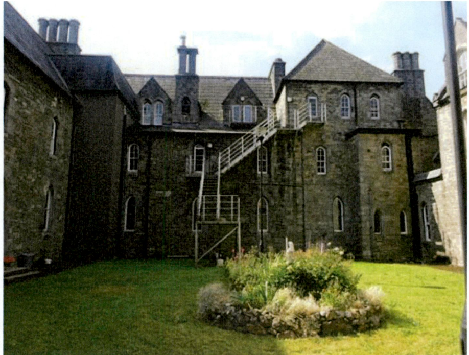
View above (E13) of the three-storey element of the southern wing alongside two-storey wings with attic accommodation.
