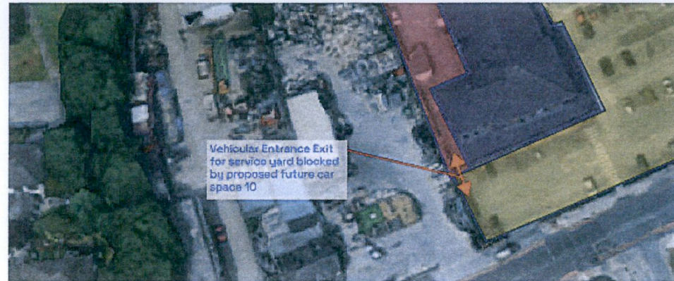
Fig 4.3 - Existing access in daily use since 1988 is being blocked by the development in an unauthorised manner
