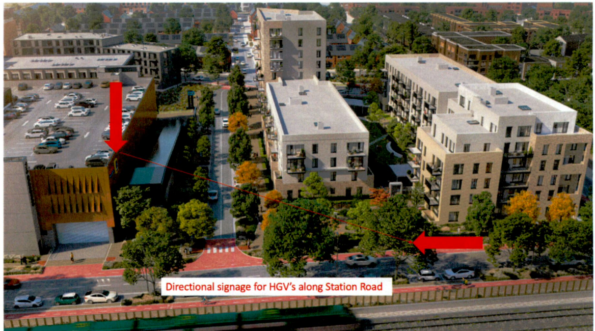
Figure 1: CGI showing positioning of directional signage placement on building in line of sight for vehicular traffic travelling along Station Road.
