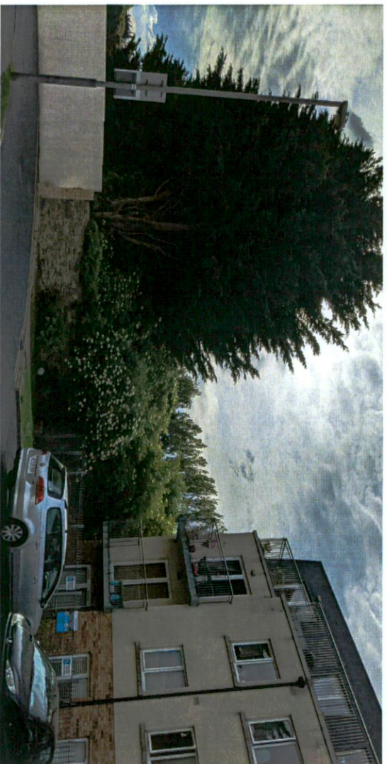
Above: View from east Eaton Drive with existing boundary wall and trees
