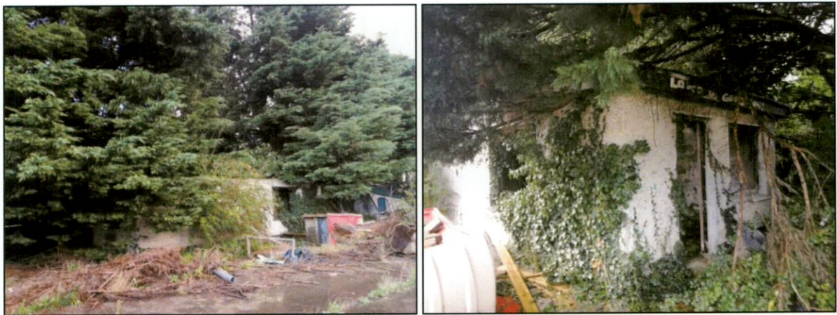
FIGURE 6. SINGLE STOREY STRUCTURE WITHIN PROPOSED DEVELOPMENT SITE.
