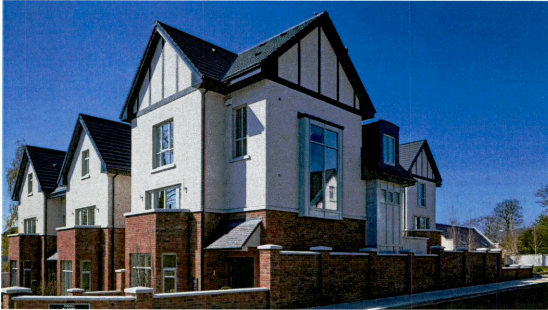
Pic 2 – 3 storey Semi Detached Houses - Source – Google Images
