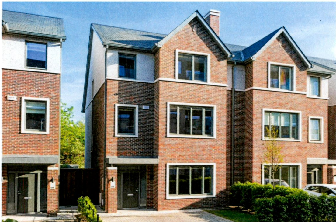
Pic 1 – 3 storey Semi Detached Houses - Source – Google Images
