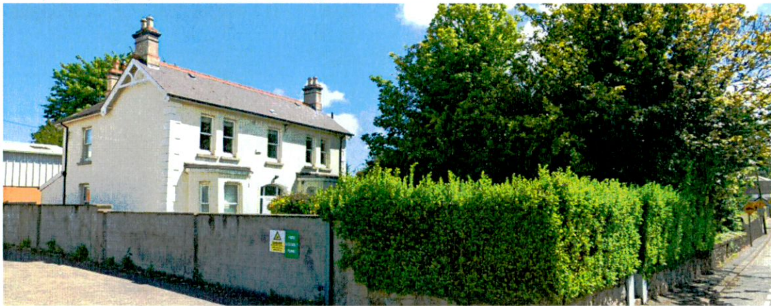
Acrebrook House immediately north of subject site – Appears as a late 19 th / early 20thC replacement of an earlier house of the same name. Rendered façade, quoins, ground floor bay sash windows, natural slate roof, late 19thC aesthetic.
