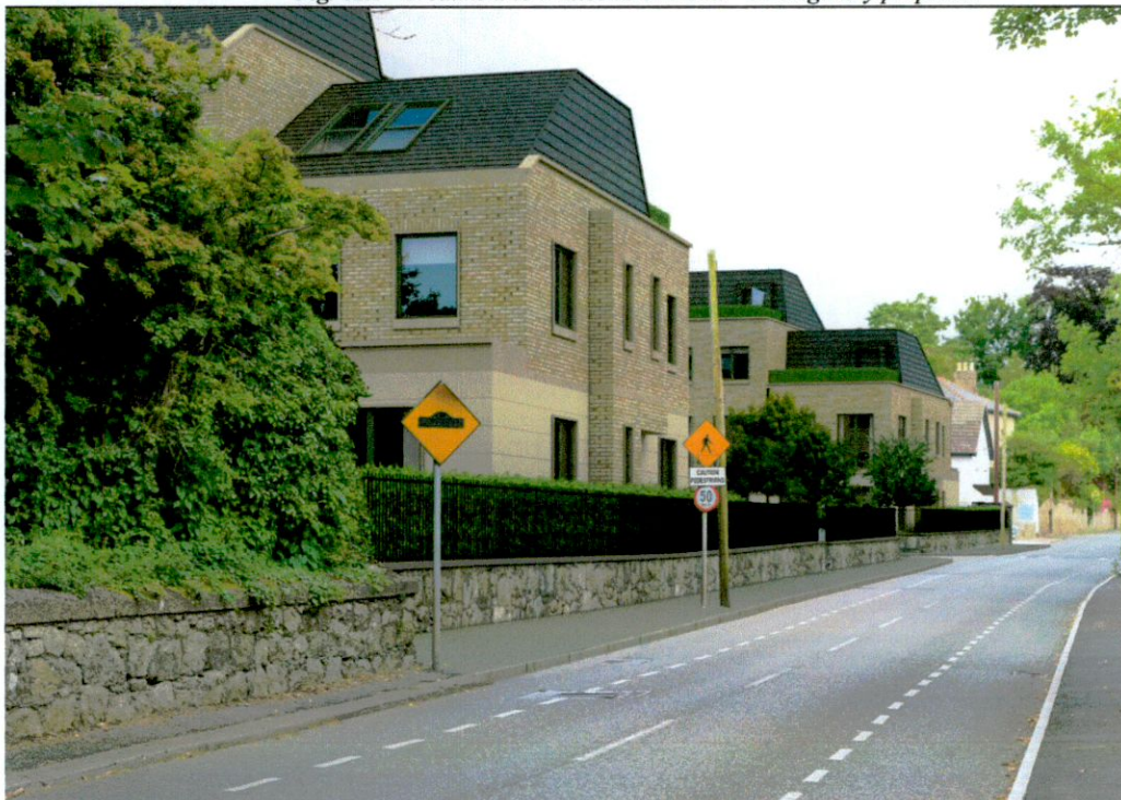
Fig. 12B –Treatment to Whitechurch Road – Gable ends create a focus and anticipation of the central amenity space. Additionally the two units along the road have been reduced in scale by one floor to improve the massing of the ensemble as encountered along the road.
