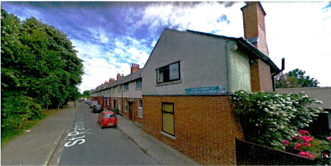
St. Patrick's Cottages behind the Mill House – 2 storey early 20 th C Brick ground floor, render above, natural slate roof, painted window frames.
