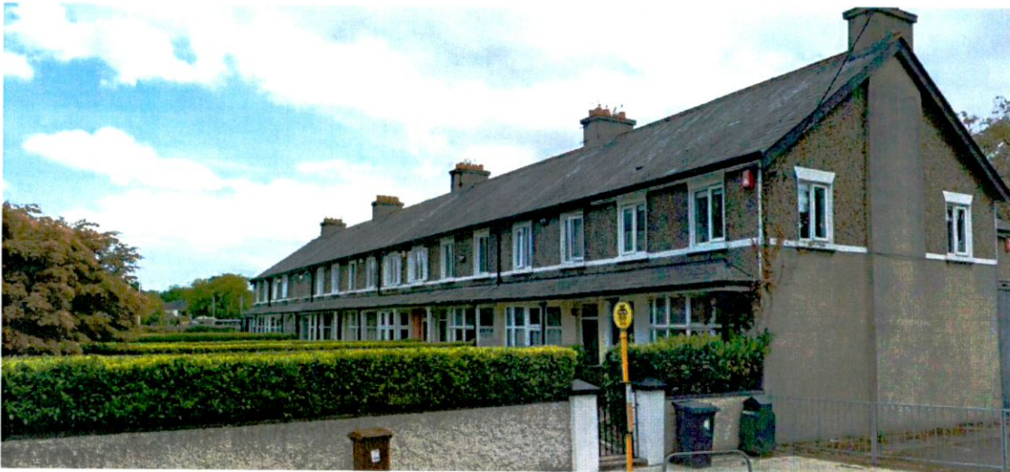
At the northern end of Willbrook adjacent to the Church, perpendicular to the road with rear parking 8 houses Early 20thC: drydash render, painted string course/ lintols/ windows, natural slate.
