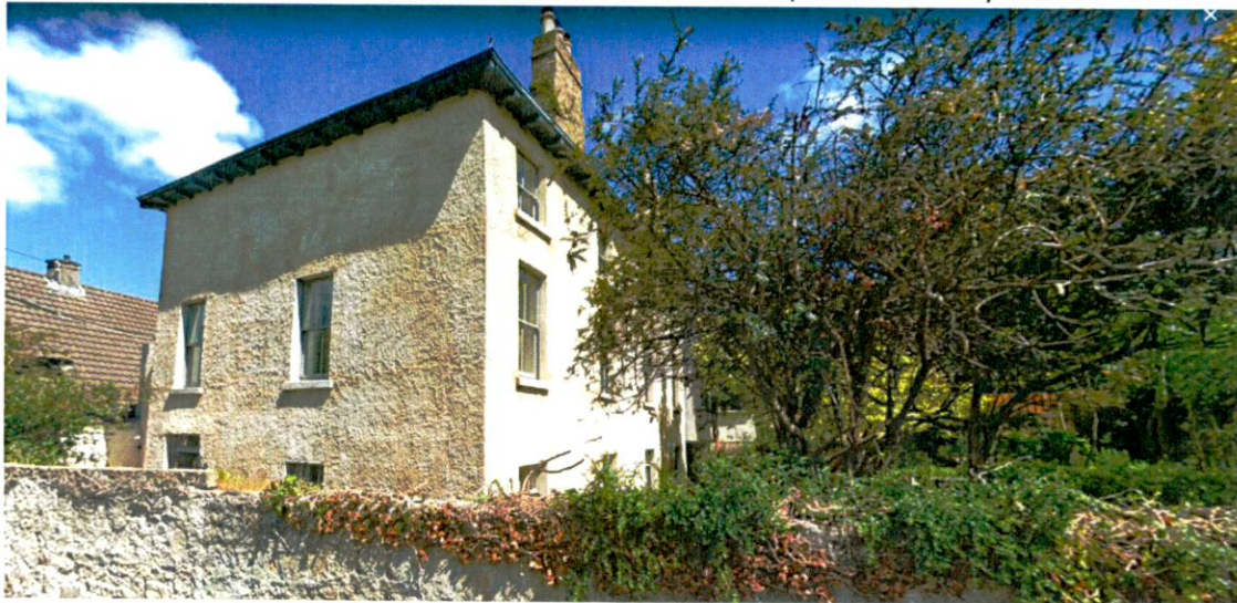
The Mill House Protected Structure – above & below
