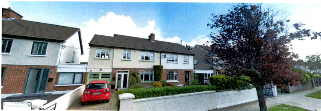
Grange Park Estate – Further South of ACA on Whitechurch Road Later 20thC estate housing, brick and painted nap render with concrete tiled roofs
