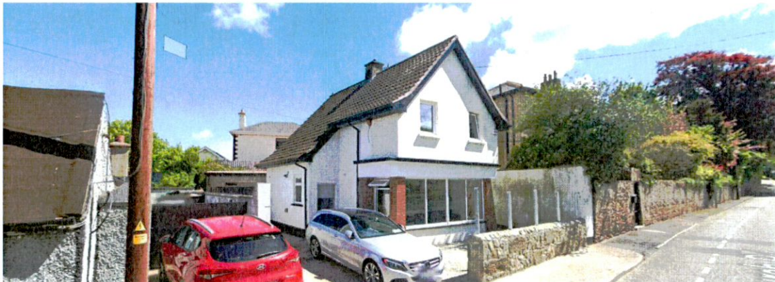
Late 20thC one-off House immediately south of subject site and adjacent to the Protected Structure on the site of the mill. Painted nap render, brick dressings, concrete tiled roof.
