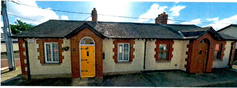
St. Patrick's cottages, single storey rendered/ painted, brick dressings, natural slate roof Tara Hill Crescent/ St. Patricks Cottages – Grange Road side of Green – Focus low density type of ACA
