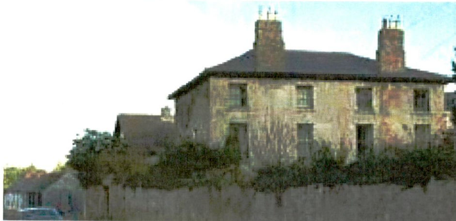
4 bay 3 storey with natural slate roof and tall chimneys with tall pots. Off-white Harling lime render façade finish with granite cills. Entrance on St. Patrick's Cottages, obscured by wall and planting.
